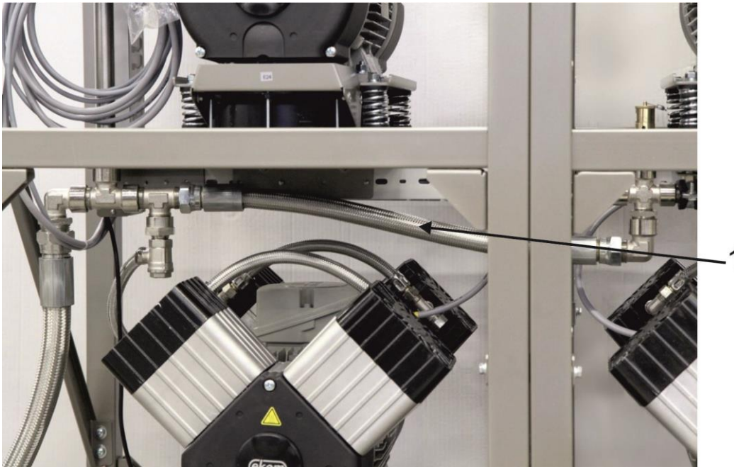
Fig. 12: Connecting the compressor modules
